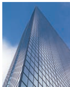
HVAC / Building Management
